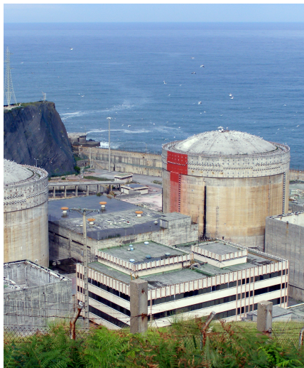
Lemoiz Nuclear Power Plant
