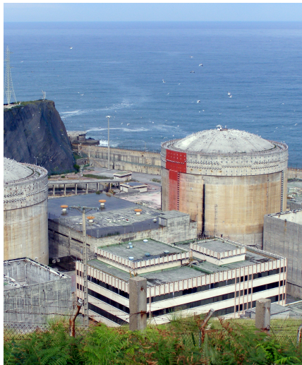
Lemoiz Nuclear Power Plant
